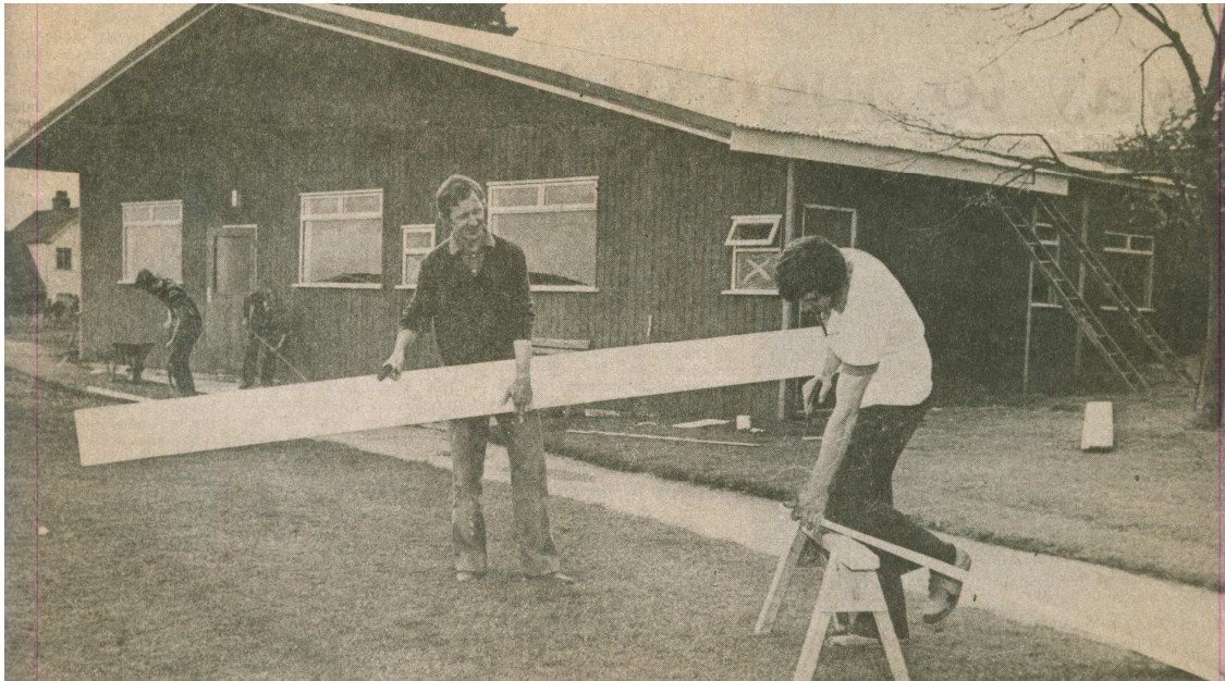
Cricket Club & Table Tennis Club members hard at work completing the building of the new Pavilion, ready to open May 1981. John Baldrey can be seen centre picture holding a plank of wood.
